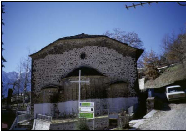
Figure 4: The deformation of the shape of the temple in Paleoselli is quite impressive, once no fractures have been observed on the walls.
