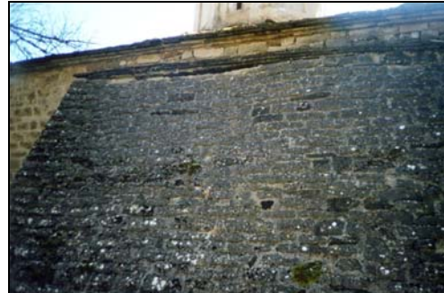
Figure 2: The detachment of the thick supporting wall from the wall of the temple on the north side of the temple
