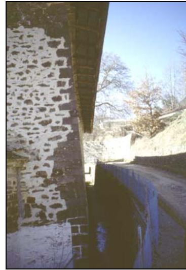
Figure 5: The northern side of the temple. The seepage is obvious, as well as the tilt of the shape.
