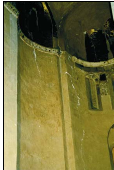
Figure 11: Fractures within the temple.
