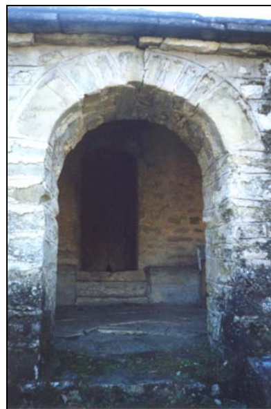
Figure 8: The entrance of the temple (north side). The fracture at the top of the span is due to subsidence on the left (northeast corner).
